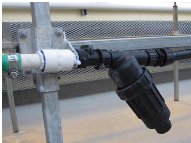
Filter for removing foreign particles in the water line
